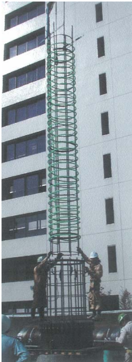
Figure 4 Construction of a Pile
