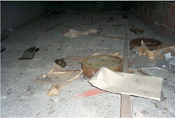
Measure 1: Insulation of the crawl roof space.
