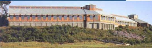
Facility HVAC Assessment, Prepared by KEEN ENGINEERING
