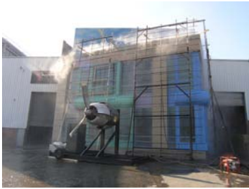
Figure 2 Dynamic Water test
