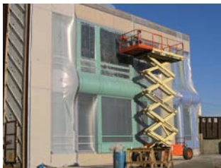
Figure 1. Lab mockup during ASTM E283 air infiltration test
