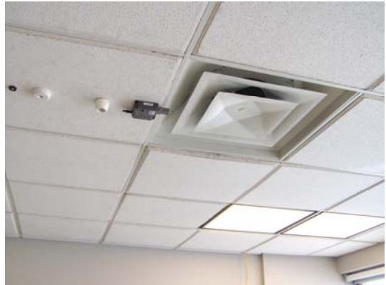
Figure B: Wireless discharge air temperature sensor used for DART demonstration.
